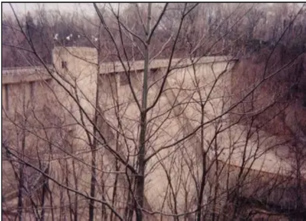
Standing at almost 90 feet high with a width of 500 feet across, the water levels at the dam's base have always been negligible. The structure, however, is used by firefighters for repelling practice during training exercises.
